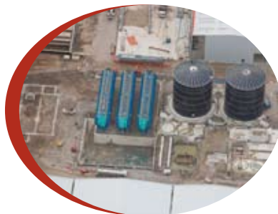
Kirk's Digester Tanks at the Lancashire Treatment Plant
